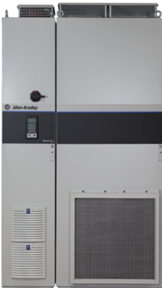
PowerFlex 755TL drive for harmonic mitigation
