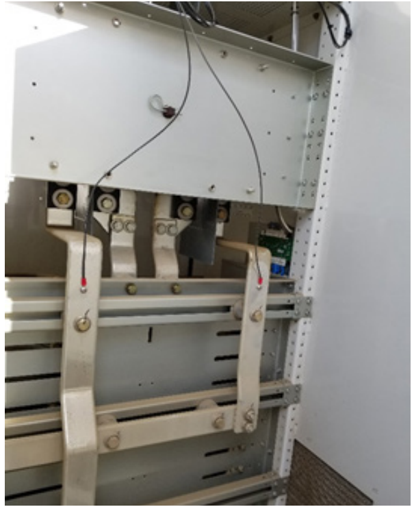
Connections at the inverter show the termination of PESD to the 1000V DC Bus.
